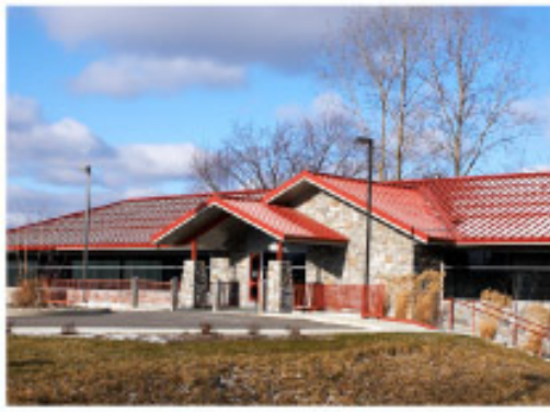
Two story structural steel commercial office building with second floor bar joist and deck mezzanine system with BattenLok standing seam roof system supplied by A G Bell for Tecton Corp., Fort Wayne
